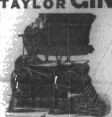
With Feeder and Condenser This Gin is an improvement on the old "Taylor" Gin, manufactured so many years ago at Columbus, Ga. It is compact, of simple construction, gins fast, and cleans the seed well; has an iron frame, is of the very
