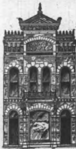
THE BANK BUILDING 1923 First Avenue.
