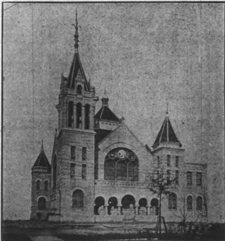
First Baptist Church, Jacksonville, Florida.
