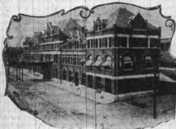
Union Passenger Station, Montgomery.
