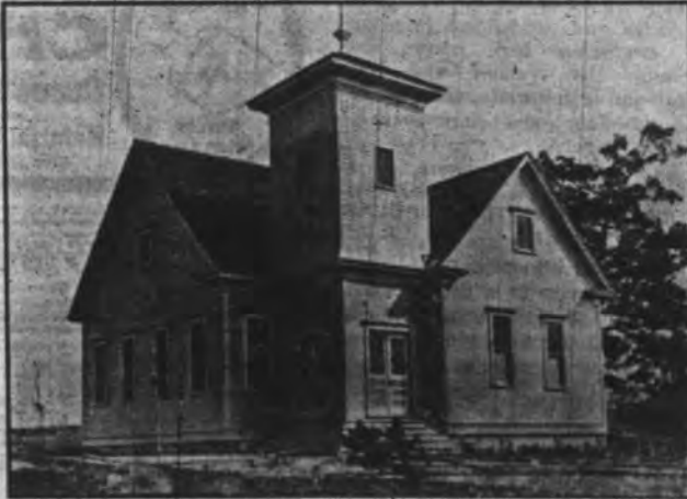
BUTLER BAPTIST CHURCH, BUTLER, ALA. Just completed at a cost of $2,500 including the seating. It is seated with circular oak pews. Butler is one of the oldest towns in the state and has never had a Baptist Church till about two years ago.
