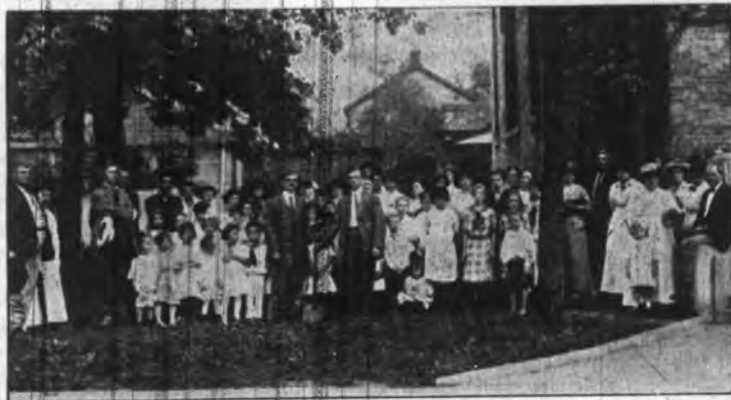
BREAKING GROUND FOR AN $8,000 ANNEX TO THE FIRST BAPTIST CHURCH OF BESSEMER—REV. M. K. THORNTON, PASTOR; MR. GWYLYM HERBERT, SUNDAY SCHOOL SUPERINTENDENT.
