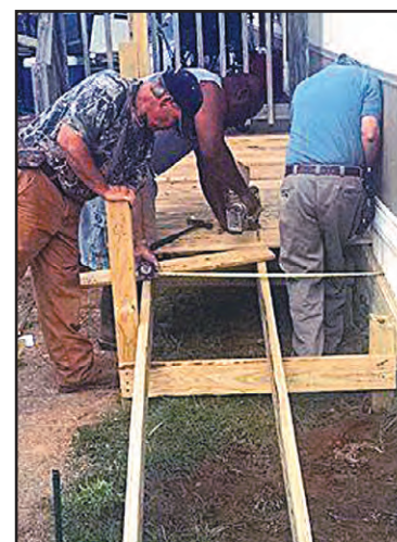
Photo courtesy of Irby Jackson Team members from Crestline Baptist Church, Tuscaloosa, work on a ramp for 12-year-old Mylan Marks during A Day of Hope.
