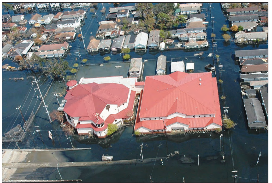
Franklin Avenue Baptist Church, New Orleans, Louisiana
