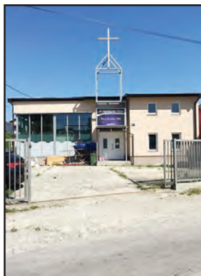
Photo courtesy of Jay Stewart Dubrava Baptist Church continues to grow and has planted two churches with help from missions partners.
