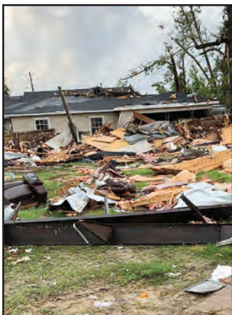
Facebook photo An EF-2 tornado caused extensive damage in East Brewton in Escambia County on June 19.
