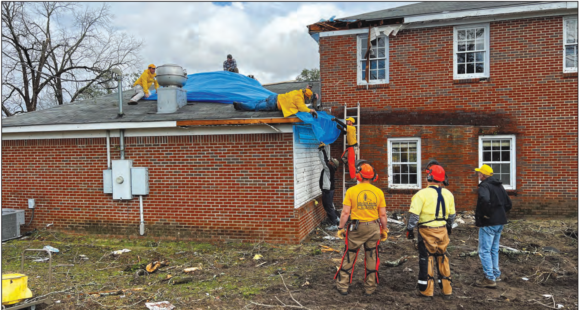
Photo courtesy of John Thomas Alabama Baptist Disaster Relief vol- unteers tarp a roof at FBC Cottonwood after a tornado damaged the building Jan. 9.
